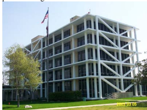
Figure 4. The city hall of Costa Mesa, a nonductile concrete building retrofit with an external steel frame. The city hall is being instrumented under CISN to confirm performance of the retrofit technique, and to provide information on appropriateness for occupancy during response activities after the event.
